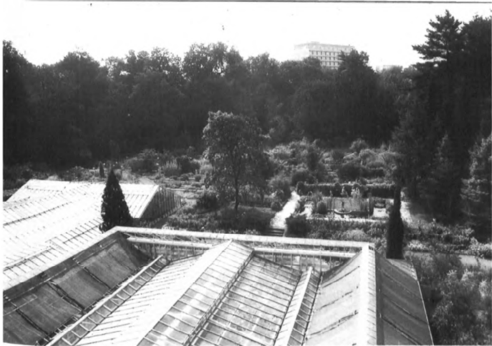
Glass house and general view
